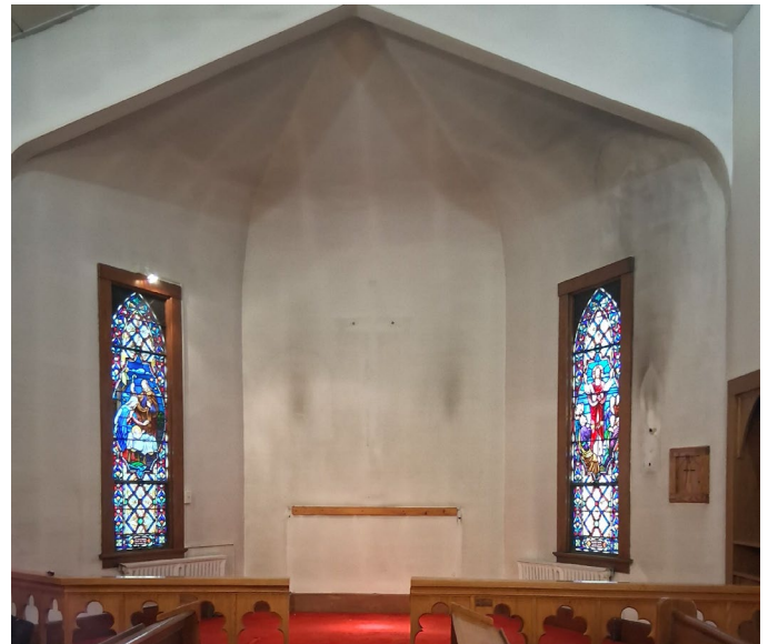
Our Sanctuary before cleaning, repairs and painting were performed.
